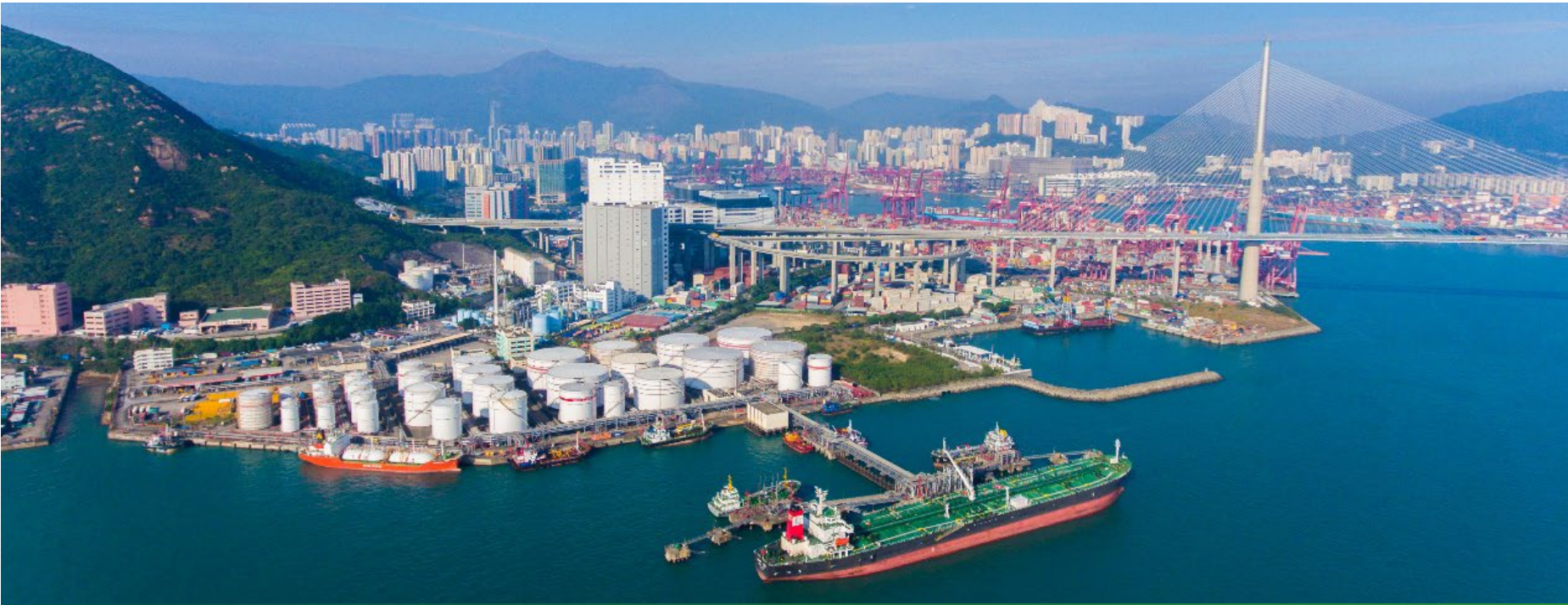
Hong Kong Sinopec Oil Terminal at Tsing Yi, the largest single oil terminal in Hong Kong
