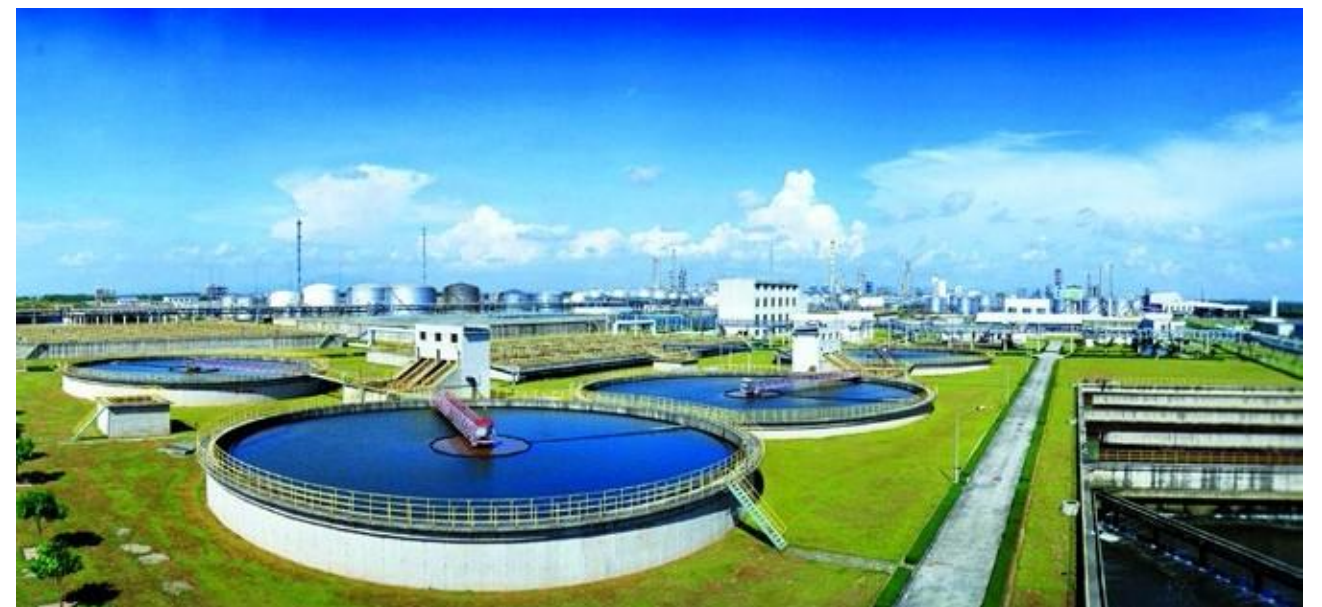
The ethylene effluent disposal plant owned by Sinopec Maoming Petrochemical Company
