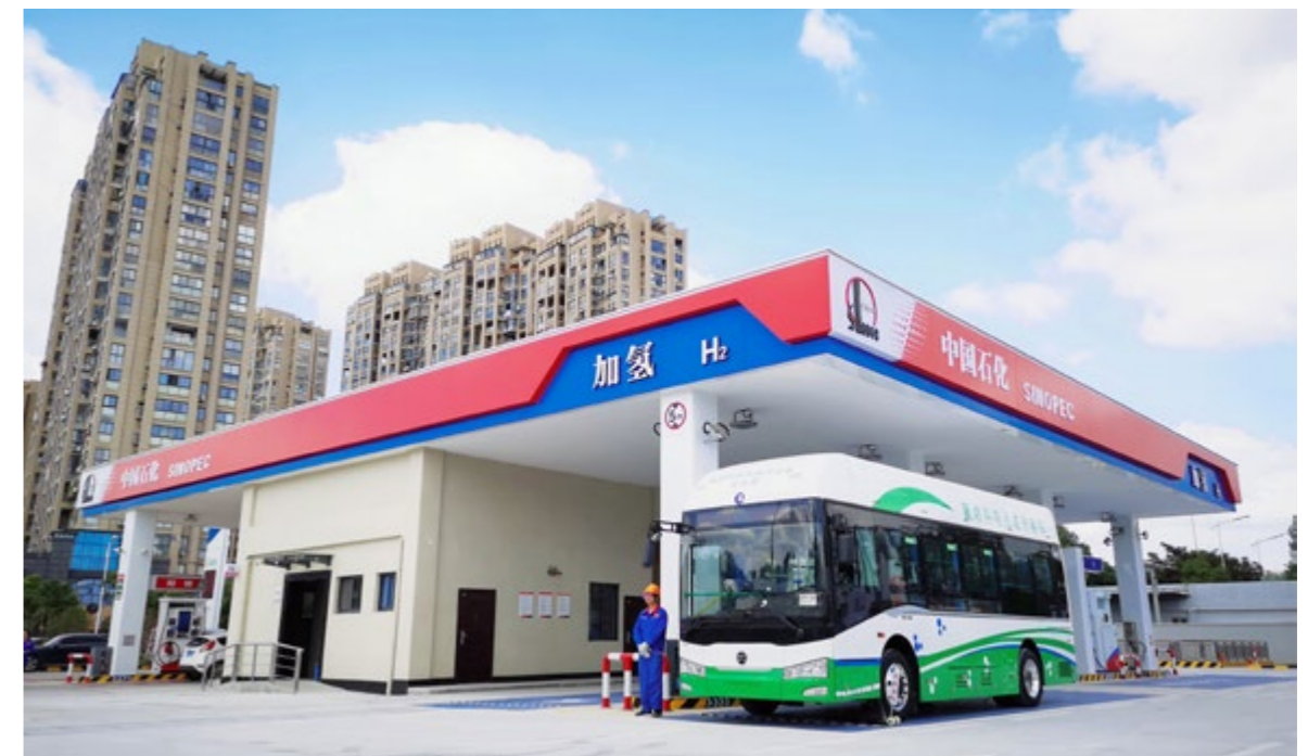
Hydrogen refuel station in Jiaxing, Zhejiang
