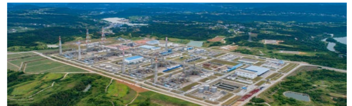
Sinopec Corp. built China's first large-scale natural gas purification plant in Yuanba Gas Field
