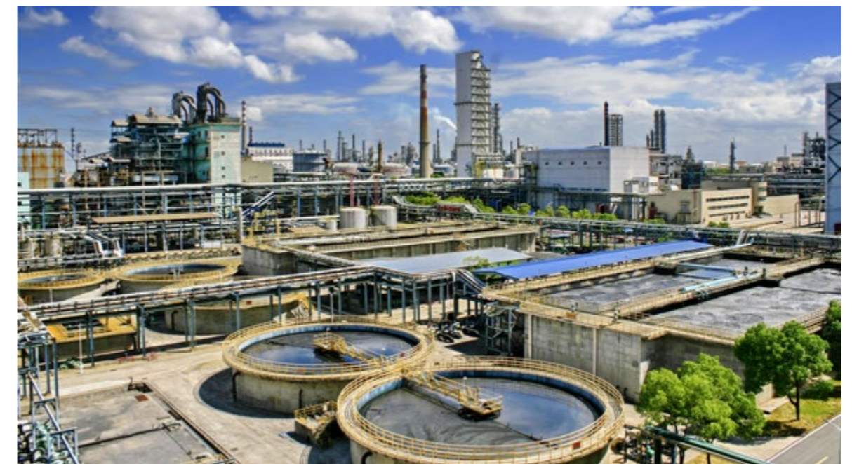
Sewage Treatment Plant of Sinopec Jiujiang
